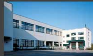
Production facility in Wetter-Volmarstein
